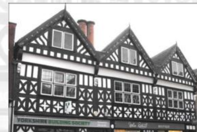
21 & 23 High Street (plastered over).
