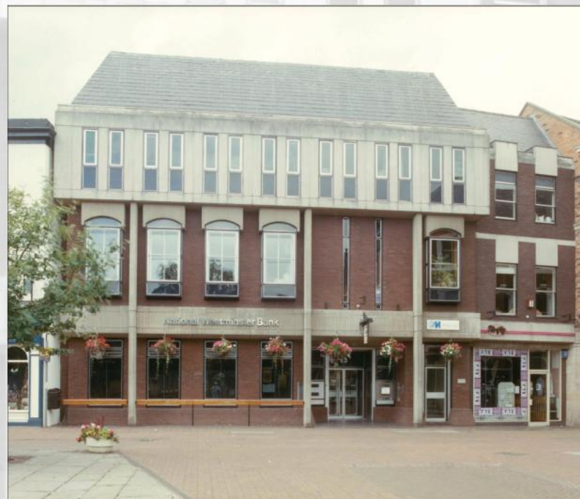
Exterior of Nantwich 36 High Street branch of National Westminster Bank plc, 15 August 1993 (Reproduced with kind permission of NatWest Group plc (Photograph ref: D7269))
