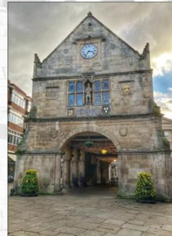
The Old Market Hall in Shrewsbury. The market halls in Nantwich would have been constructed to a broadly similar design, with an arched market place, and court rooms above. (Photo: Ian Short)
