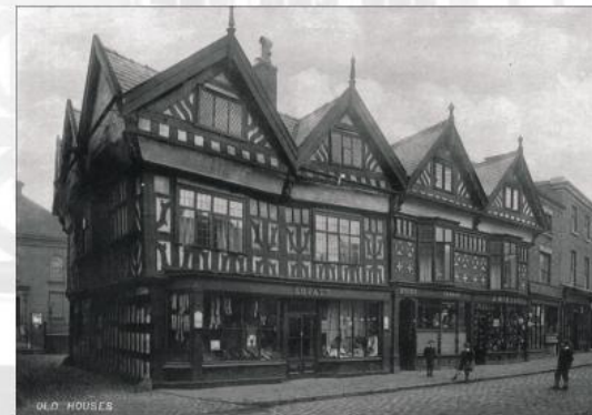
46, 44 & 42 High Street (plastered over).
