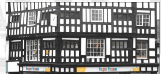
Regent House (Hope House), at the Junction of High Street with Swine and Oat Market.
